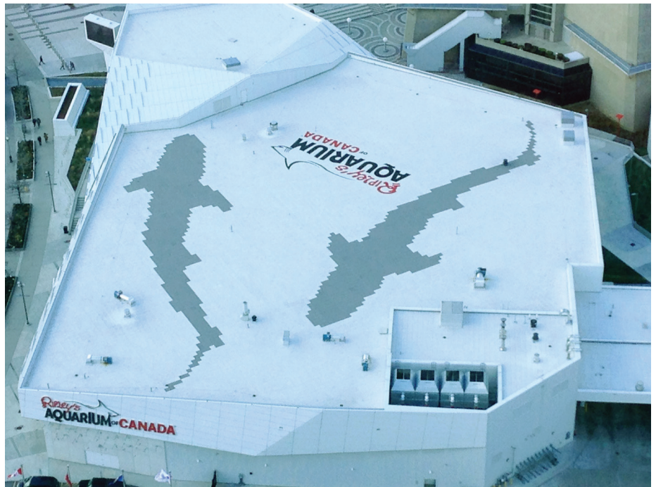
TORONTO, ON - CREATIVE DESIGN WITH SOLAR REFLECTIVE ROOF BALLAST SLABS AND CHARCOAL SLABS TO CREATE THE SHARKS
