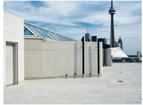
TORONTO, ON - ROOF BALLAST SLABS
