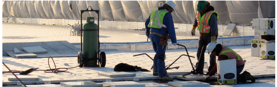
PLACING A SLAB USING LIFTING CLAMP
