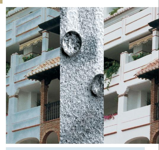
**The problem with conventional exterior paints:** The soiling of the façade becomes increasingly visible over time. On weather exposed sides in particular, microorganisms find an ideal environment for colonization in the form of adequate moisture and nutrients from dirt deposits.
