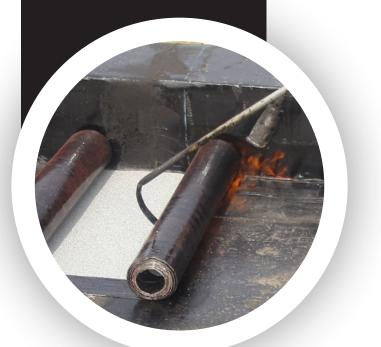
When used with a cap sheet, **Torchflex TF-95-FF-Base** satisfies the requirements of CGSB-37.56-M, as well as ASTM D6163 for Type I, Grade S materials.
