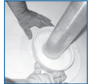
2. Ensure proper fit of 2 piece TPO Molded Sealant Pocket
