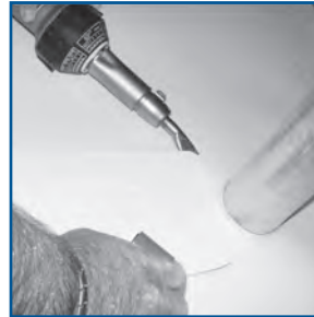
1. Overlay cut in TPO Membrane
