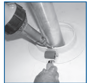
4. Heat weld 2 piece TPO Molded Sealant Pocket to TPO Membrane
